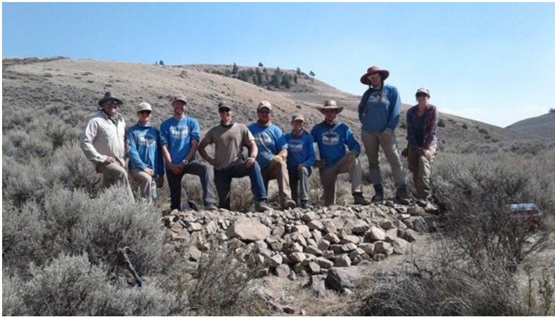
Justin Stone (USFS), Hanna Wigginton (BLM), and Western Colorado Conservation Corps members stand on a filter dam, constructed to catch runoff from a gully and reconnect a meadow system.
